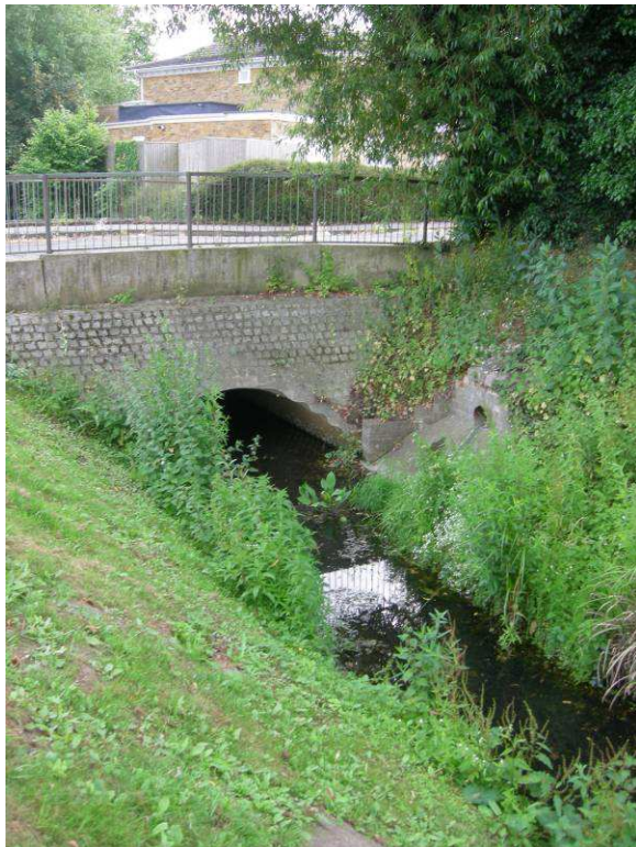
Figure 3-6 Bridge over channel, Watermans Way
