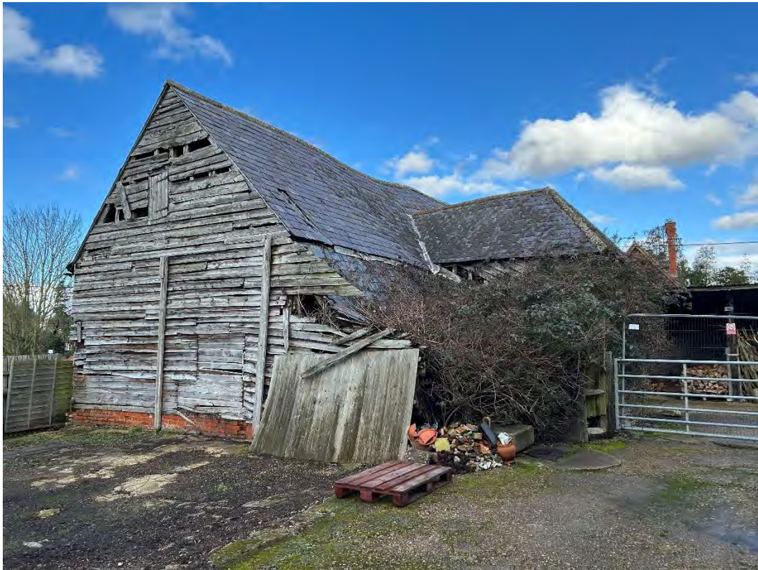
Plate 10 - Threshing Barn viewed from south
