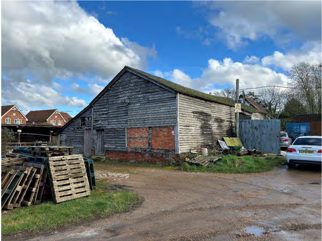
Plate 13 - Large Barn to north-west of Hatch Farmhouse, view looking west
