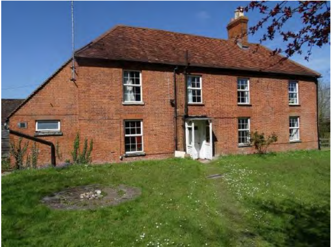
Plate 5 - Hatch Farmhouse - south-eastern elevation (in 2016/2017 sales brochure 12 )
