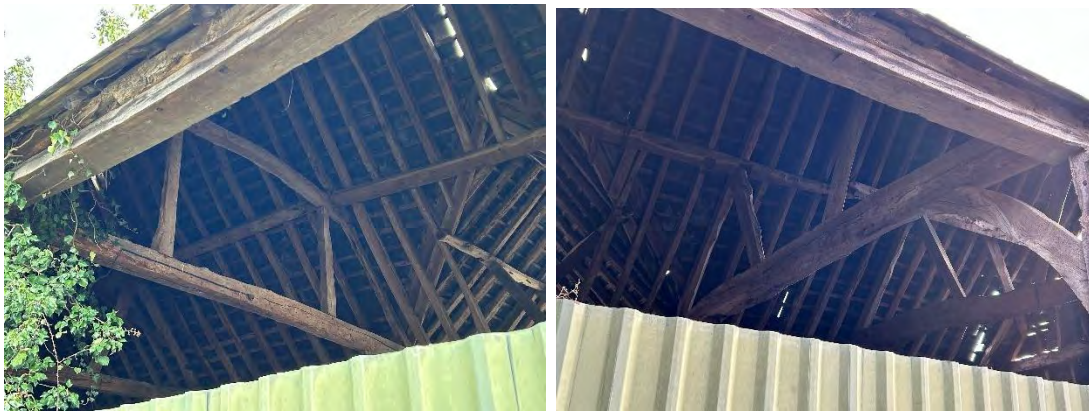
Plate 11 - View of interior of Threshing Barn with combination of queen struts (left) and raking struts (right)
