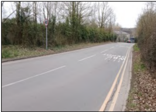
Photograph 19: Location of proposed vehicle barrier.
