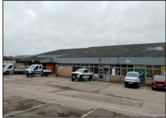
Photograph 2: Building B2, northern elevation.
