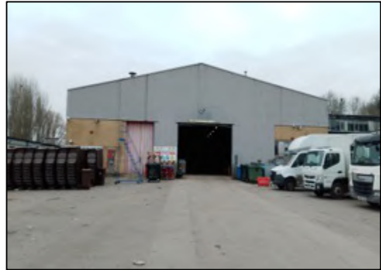
Photograph 4: Building B3, eastern elevation.
