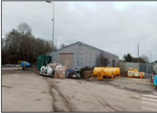
Photograph 9: Building B7, south-western elevation.
