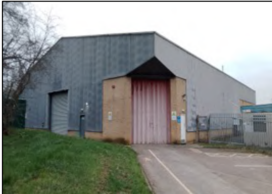
Photograph 5: Building B3, south-western elevation.
