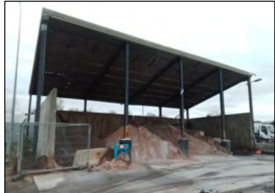
Photograph 8: Building B6, southern elevation.
