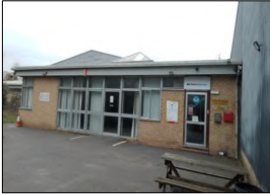
Photograph 1: Building B1, western elevation.
