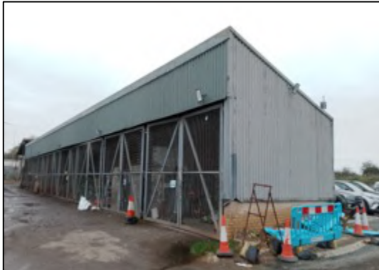
Photograph 7: Building B5, south-western elevation.
