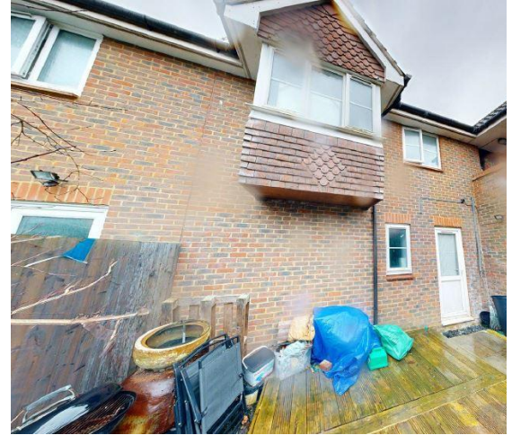
View of neighbouring roof and window
