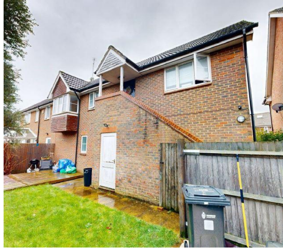
Existing Rear facade
