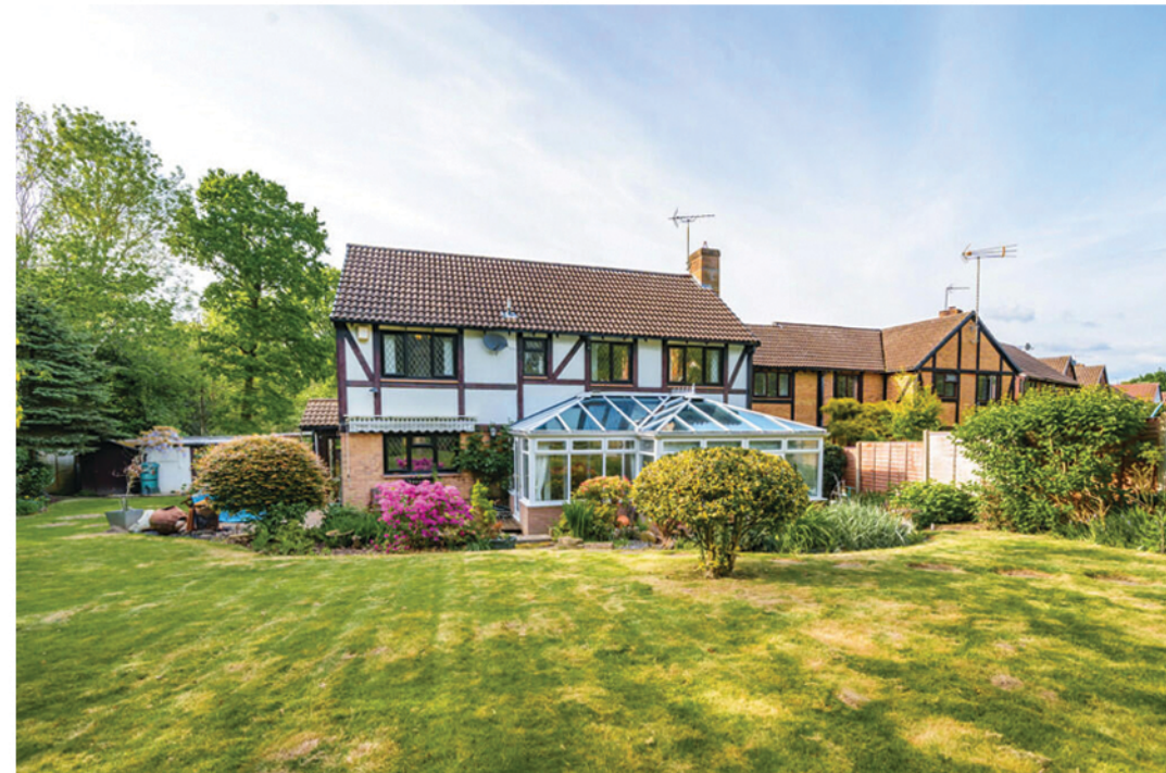
REAR ELEVATION PHOTO
