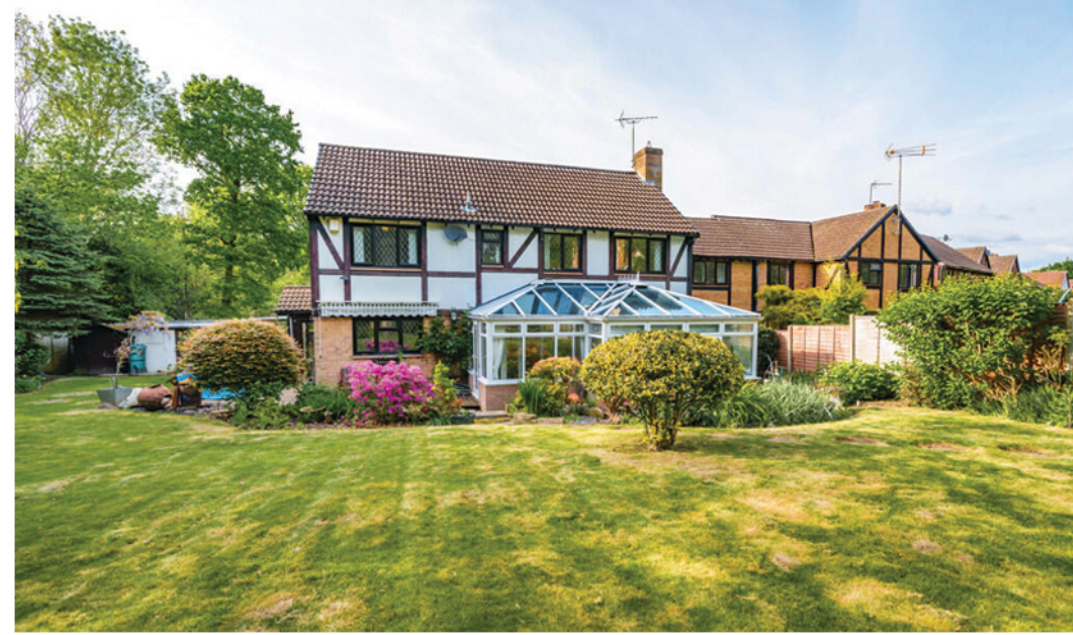
REAR ELEVATION PHOTO
