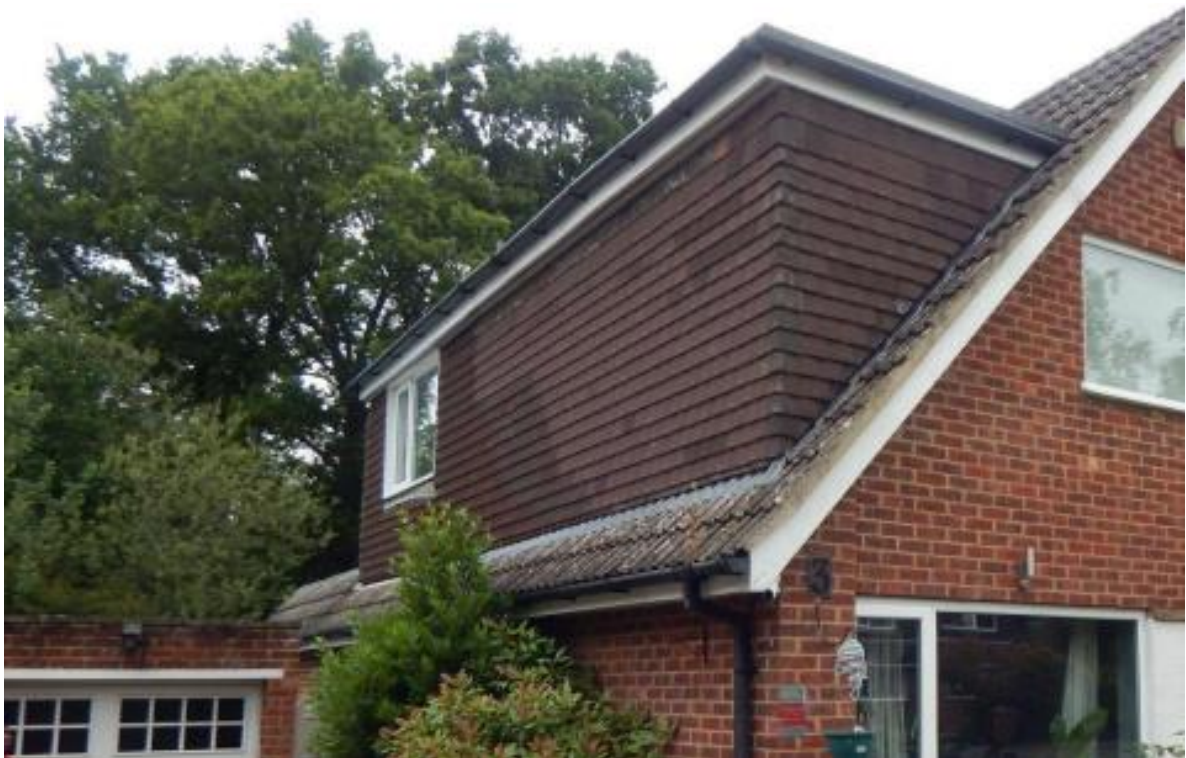
Image 5 – West facing elevation of the property
