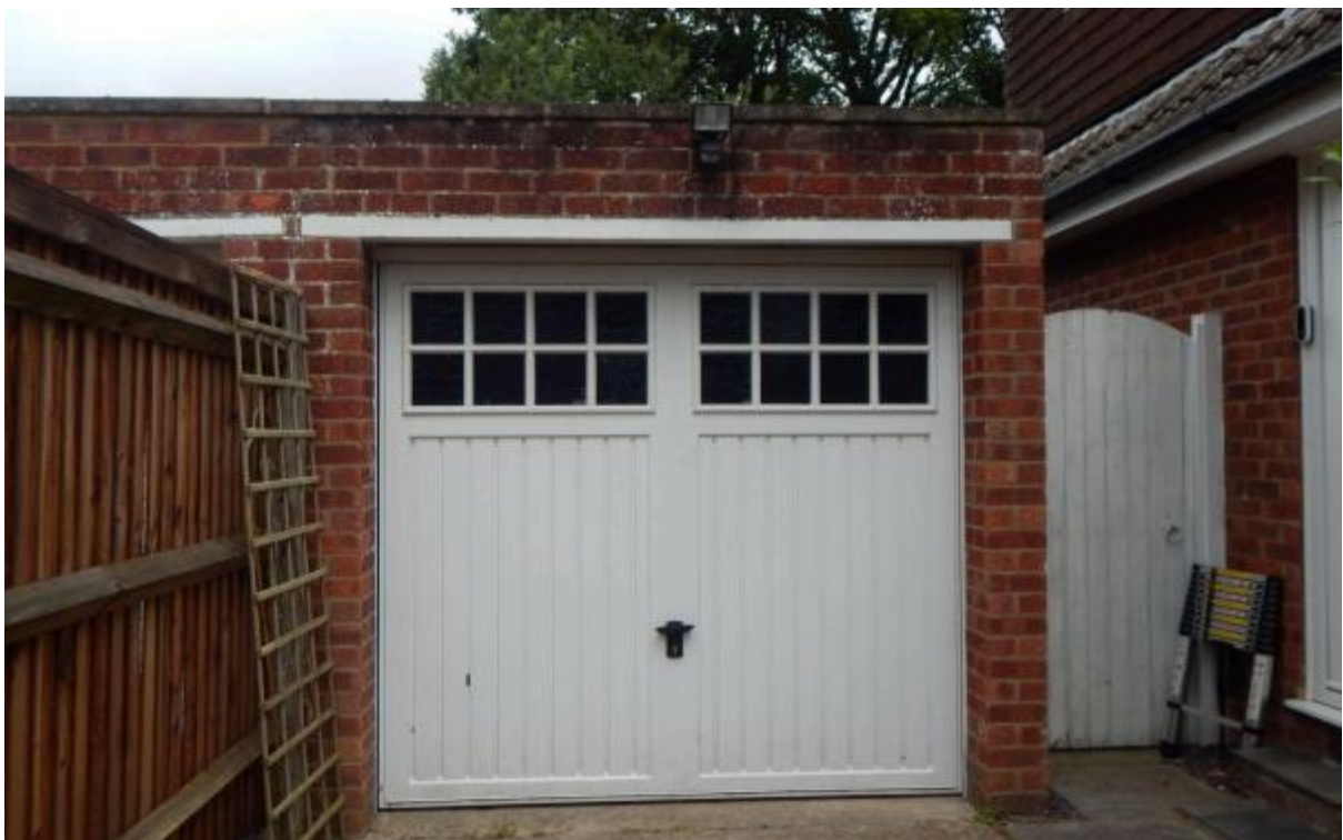
Image 8 – detached garage located to the left of the main dwelling
