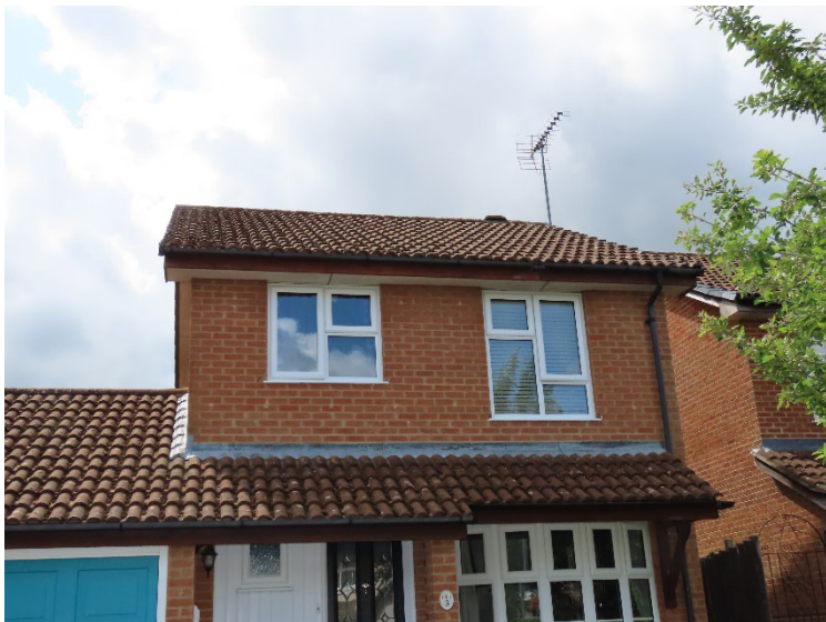
Plate 2. General view of the shed roof at the front of the property.
