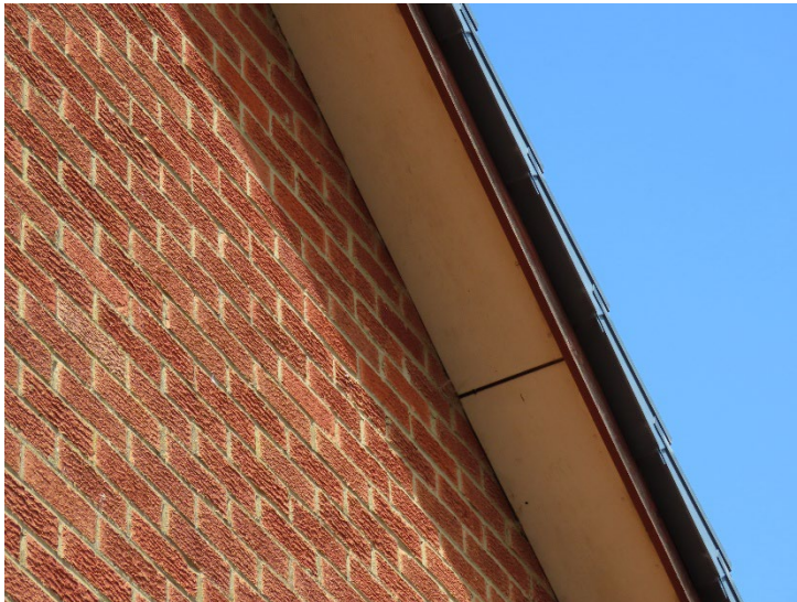
Plate 5. Typical view of the soffit and fascia.
