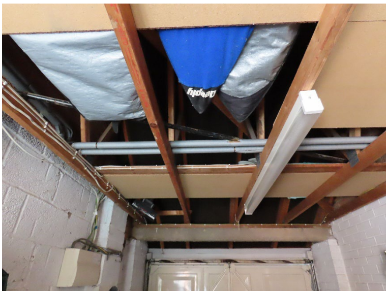
Plate 8. General view of the internal void space of the garage.
