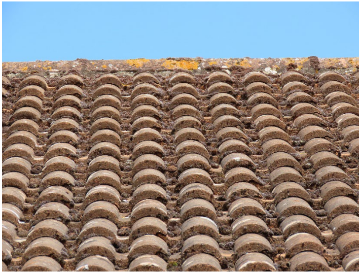
Plate 4. Typical view of the roof tiles.
