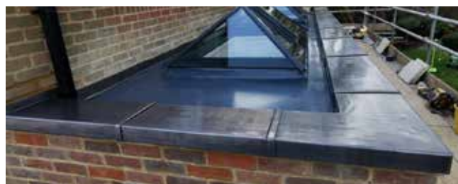
Lead capping to parapet
