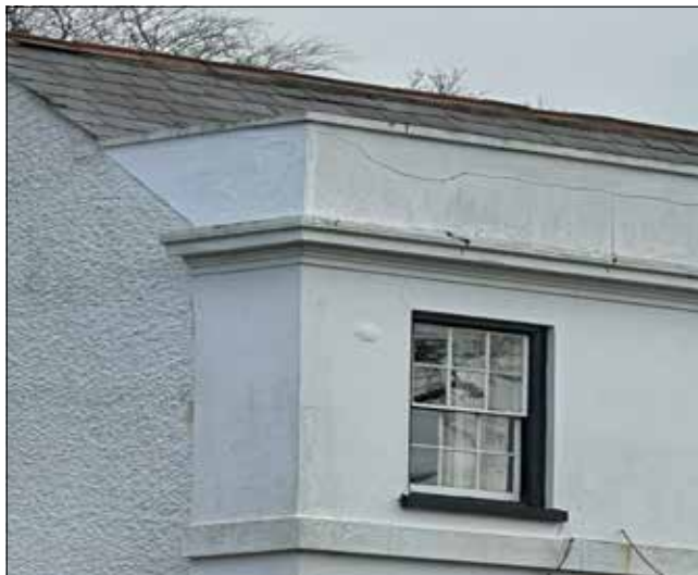
Facing Render - Existing - roughcast concrete render - white
