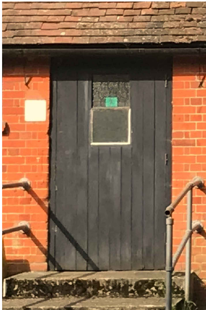
SITE PHOTO OF EXISTING SECONDARY DOOR
