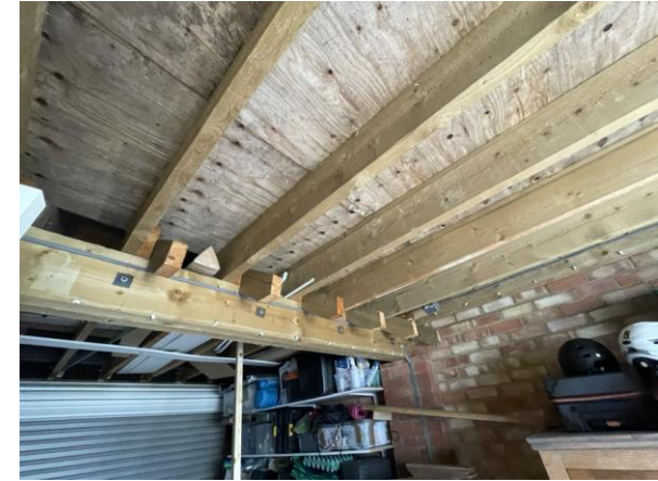
Flat roof within the garage
