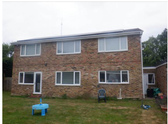
Photograph 2. Rear of property viewed from east.
