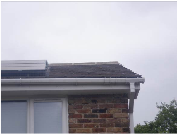
Photograph 3. Interlocking roof tiles (rear elevation).
