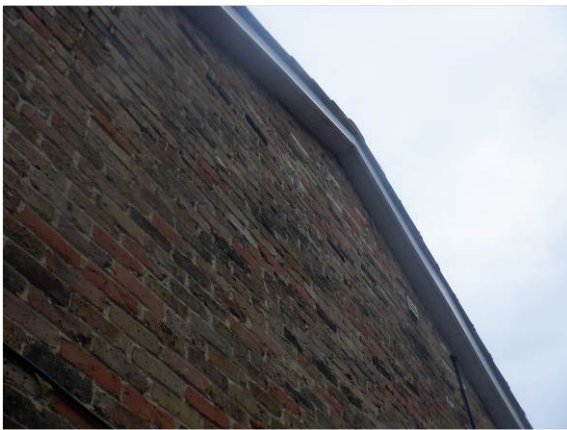
Photograph 5. uPVC soffits sealed to brickwork (northern elevation).
