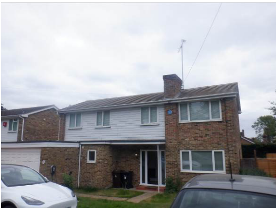
Photograph 1. Front of property viewed from west.
