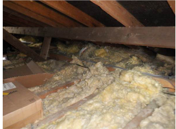
Photograph 12. Fibreglass insulation (roof void).
