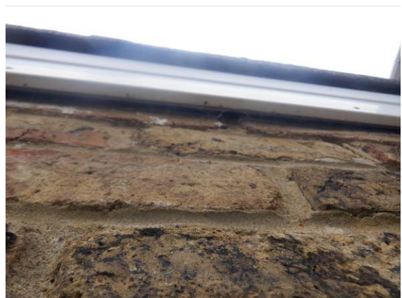
Photograph 8. uPVC fascias on single-storey garage (front elevation).
