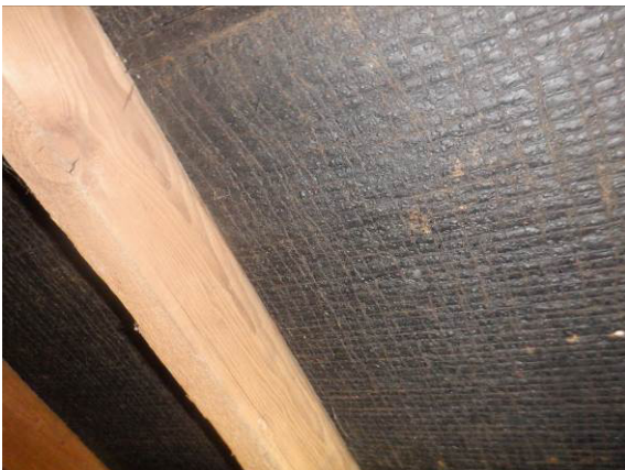
Photograph 13. Intact bitumen felt (roof void).
