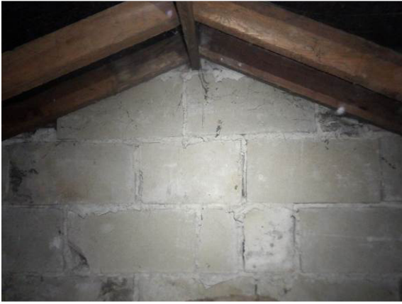
Photograph 15. Blockwork gable (roof void).
