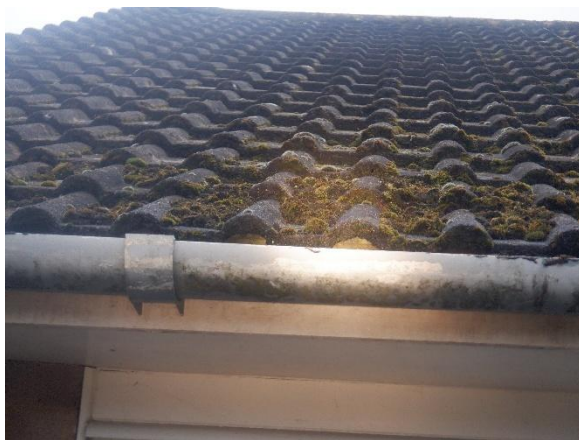
Photograph 6. Gap in mortar at the north western corner of the side.
