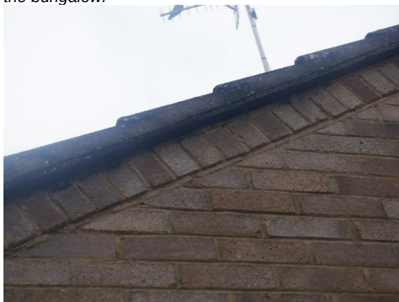
Photograph 10. Verge mortar intact at the gable end.
