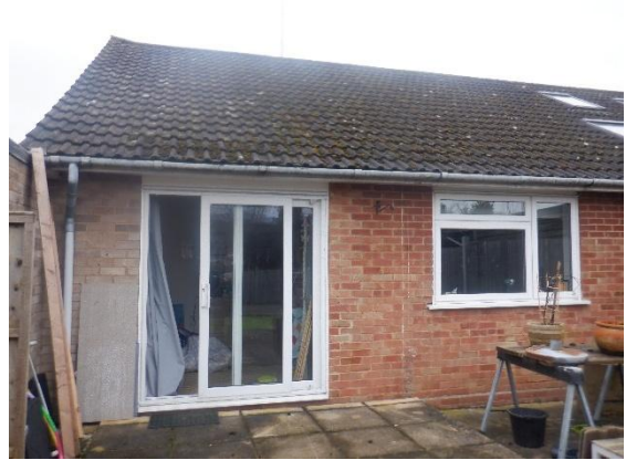
Photograph 2. Rear of the bungalow viewed from the north.
