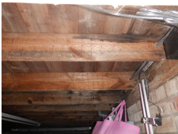
Photograph 17. Interior of the garage
