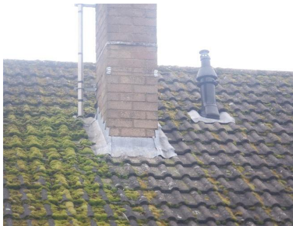
Photograph 7. Lead flashing tight around the chimney and flue pipe.
