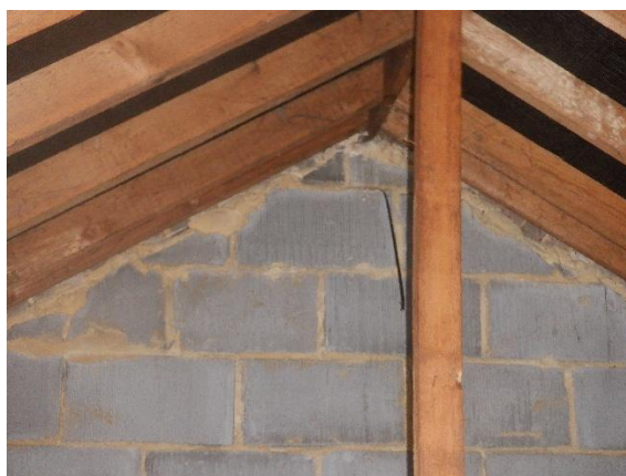
Photograph 15. Blockwork gable ends tight to felt.
