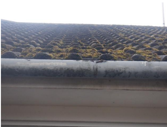
Photograph 4. Roof tiles all in place, flat and tightly fitted on the main roof.
