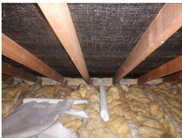
Photograph 14. Block work visible at the eaves.
