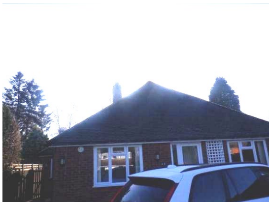
Photograph 1. The bungalow viewed from the front (north)
