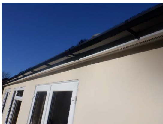
Photograph 5. Tightly fitted uPVC soffits on all elevations.
