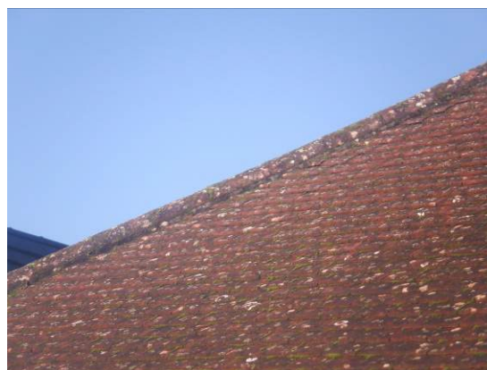
Photograph 6. The flat and tightly fitted tiles on the rear (southern) elevation with a few superficially raised tiles of negligible bat roost potential.
