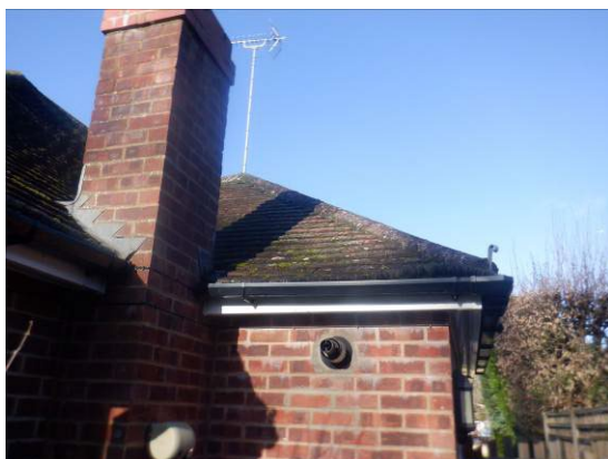
Photograph 3. The bungalow's eastern side showing the existing extension and associated chimney
