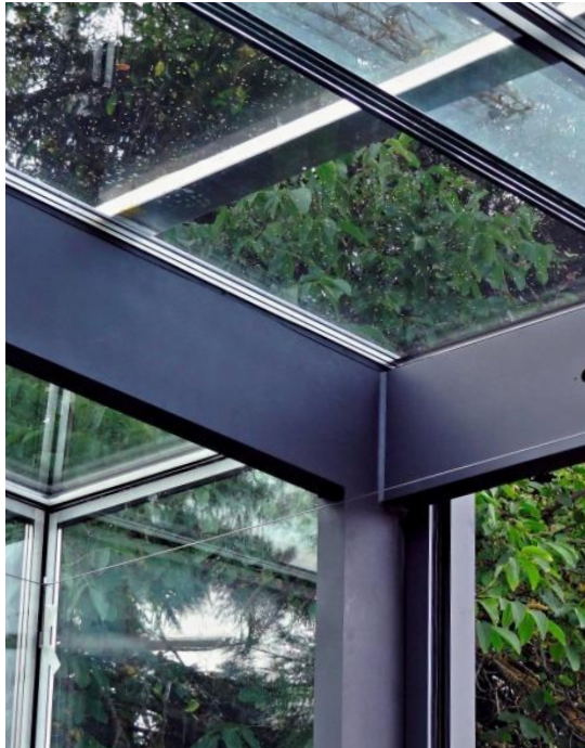
Figure 11: STRUCTURAL FRAME RAL 7021 Black Grey Slender dark-finished metal frame
