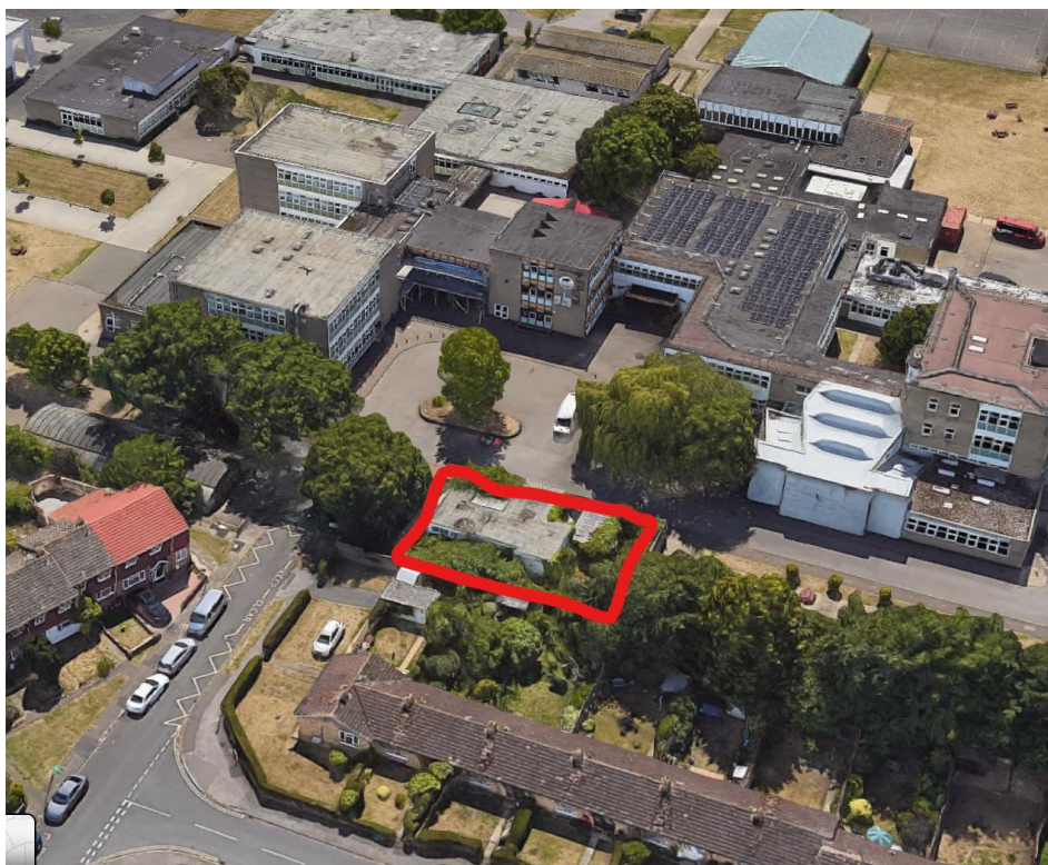
Figure 1 - Google Earth Image showing the Bungalow in context with adjoining housing and the school site
