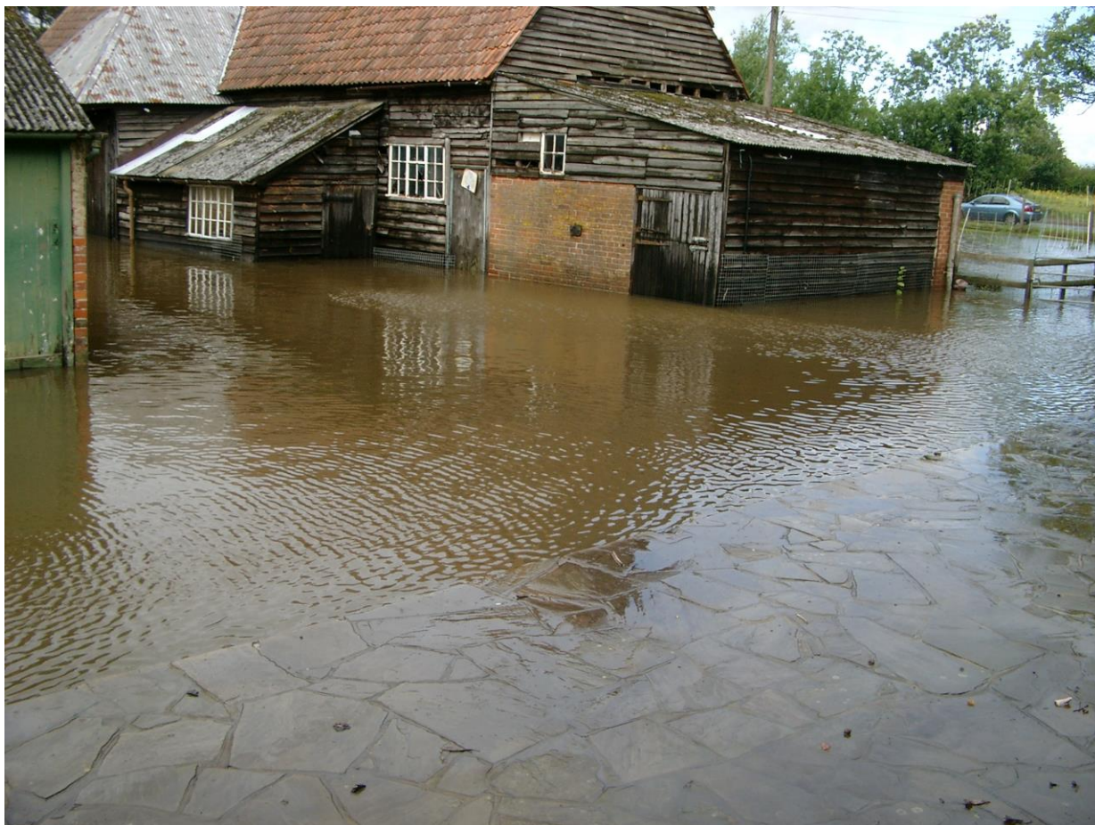
DRIVEWAY TOWARDS POND
