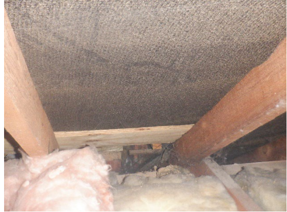
Photograph 12. Brickwork and timber visible along part of the western eaves.
