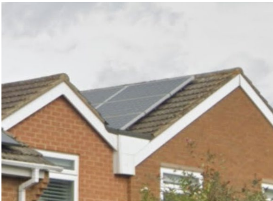
Photograph 3. Tight roof tiles at the southern side of the house.
