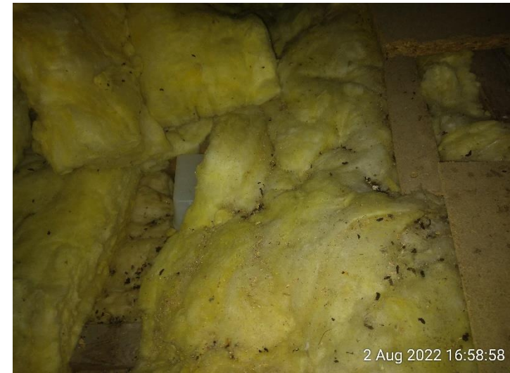
Figure 4. (above) Droppings within void 1 B1.
