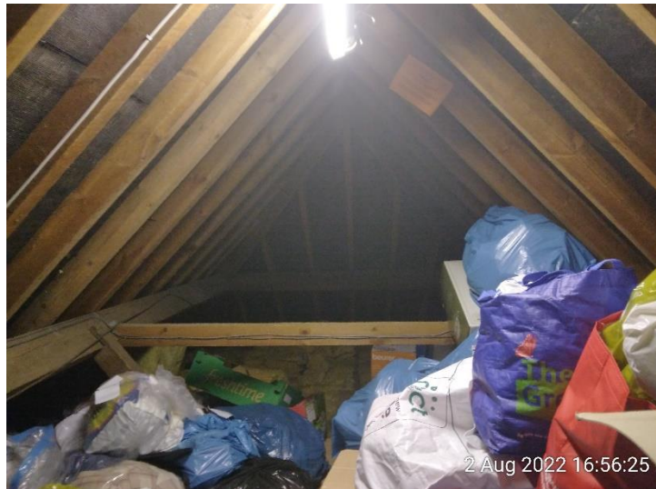
Figure 3. (above) Loft void 1 (southern) interior roof structure of B1,
