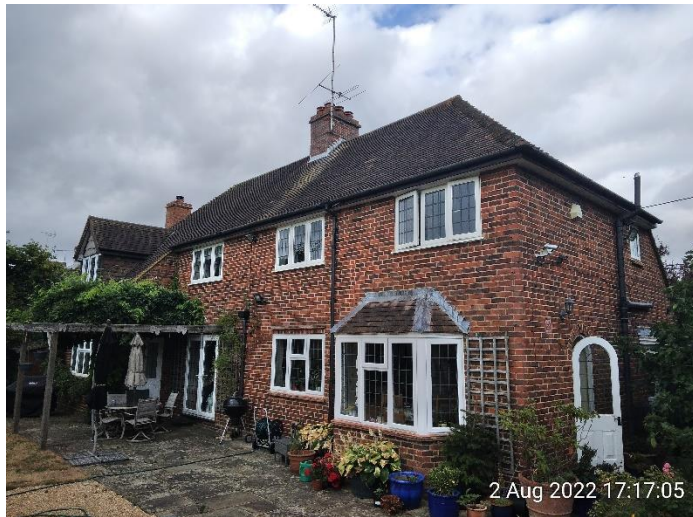
Figure 1. (above): western and southern elevations of B1.
