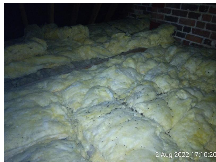
Figure 6. (above) Droppings within the loft void 2 of B1.
