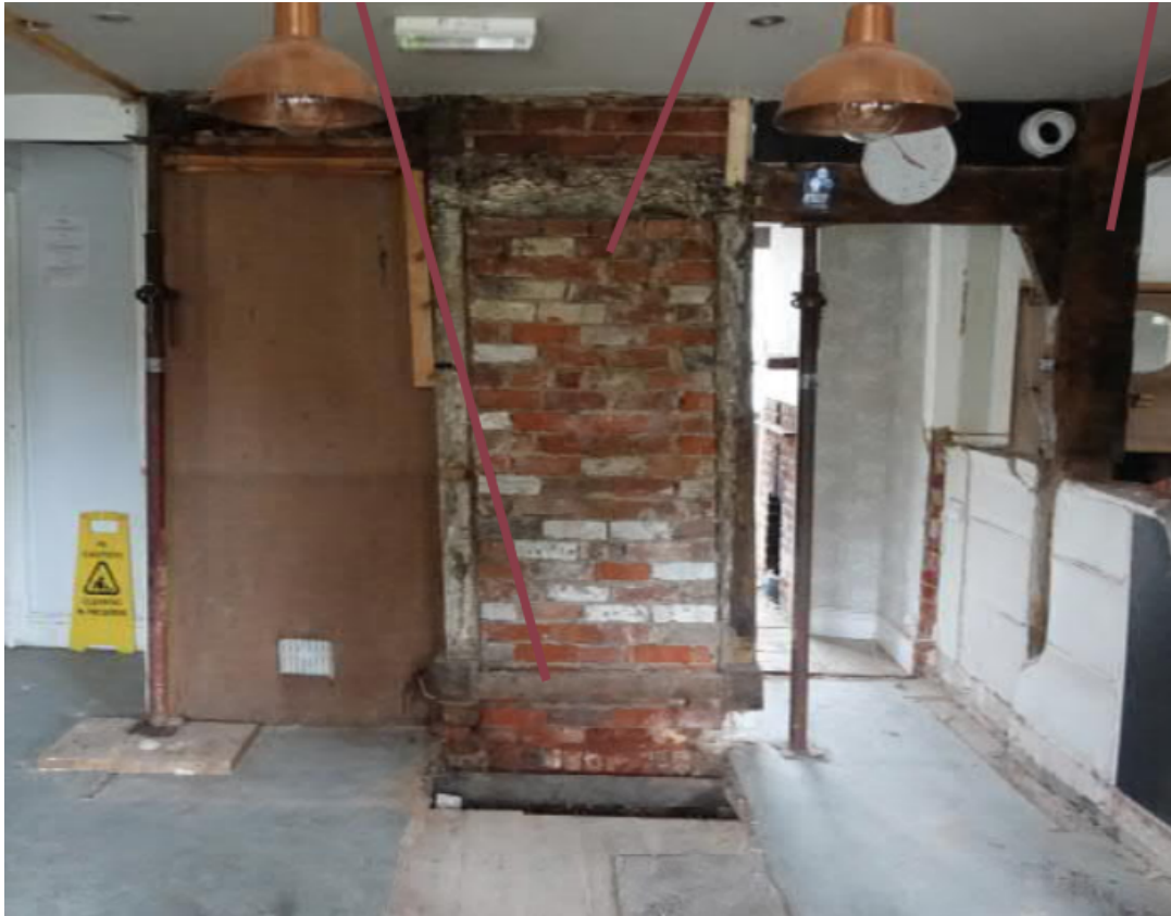
Historic blocked-up doorway – void in front suggest cellar maybe below.
