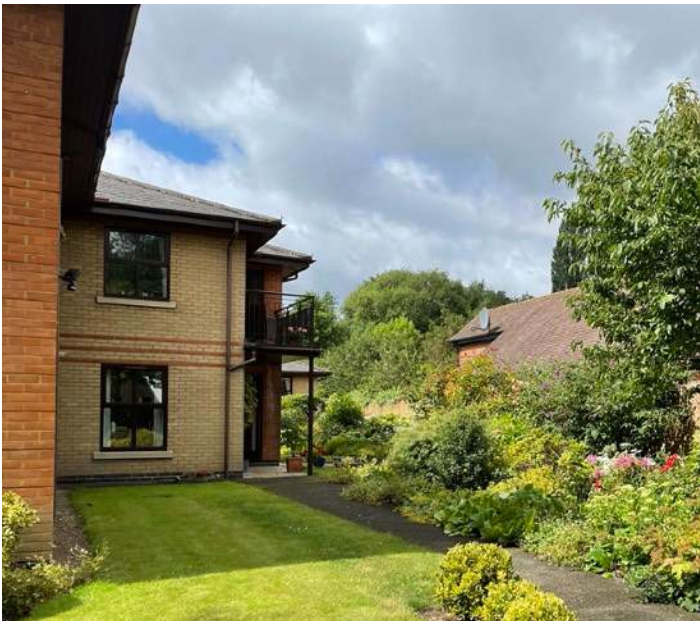
Existing Site Photo Block C to Remenham Row
