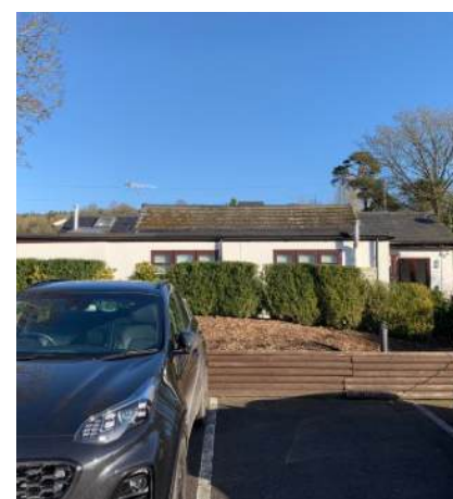
8. Lodge building now in use as a two bedroom residential unit
