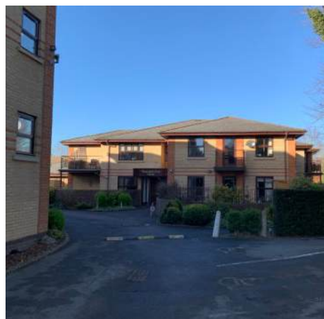
6. Access road through to service yard.
