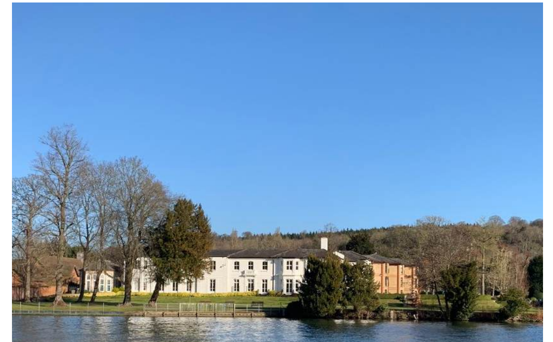
3. Looking North-East across the river to the site (winter view). The existing buildings sit behind interspersed trees along the river frontage, with the continuous range of densely wooded hills behind.
