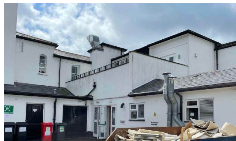
7. Rear extensions to the main house, accommodating kitchens laundry and boilers.
