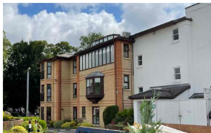
6. Rear of the 1995 block seen against the adjacent rendered stair and lift core.
