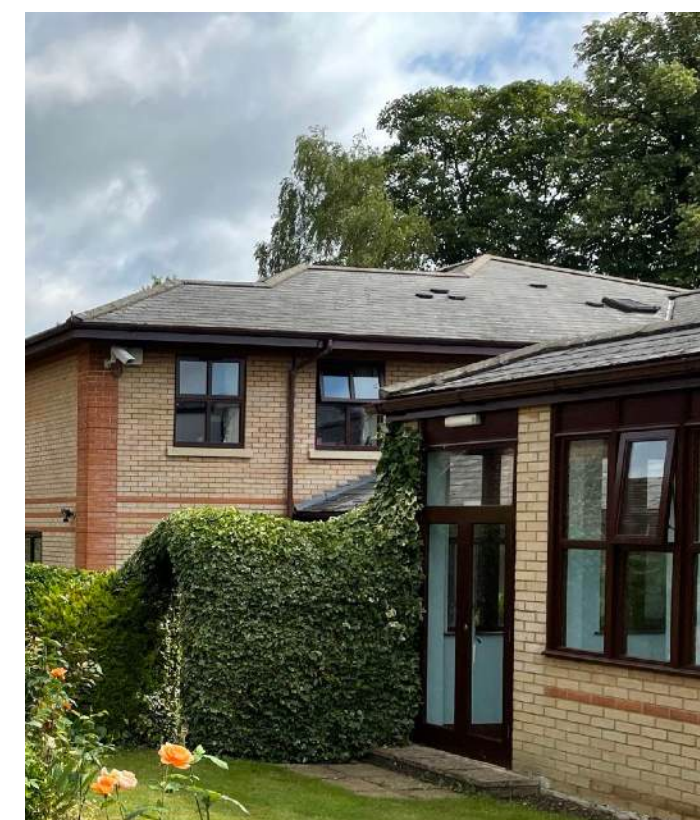
Existing Site Photo Retained Block D
