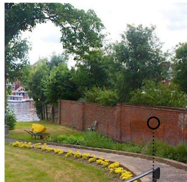
North Boundary Wall, Thamesfield
