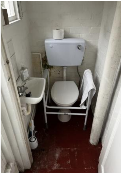
Existing ground floor WC
