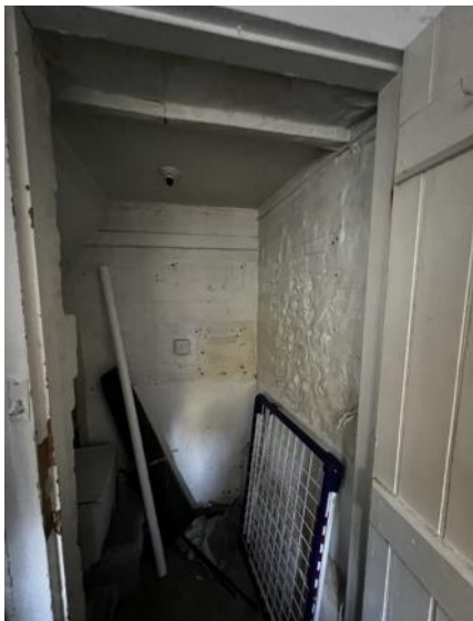
Existing under side of staircase
