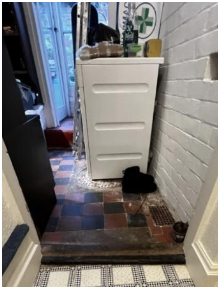
Floor finish and view to courtyard
