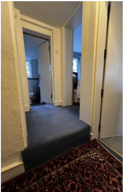
Existing steep step into rear bedroom and bathroom
