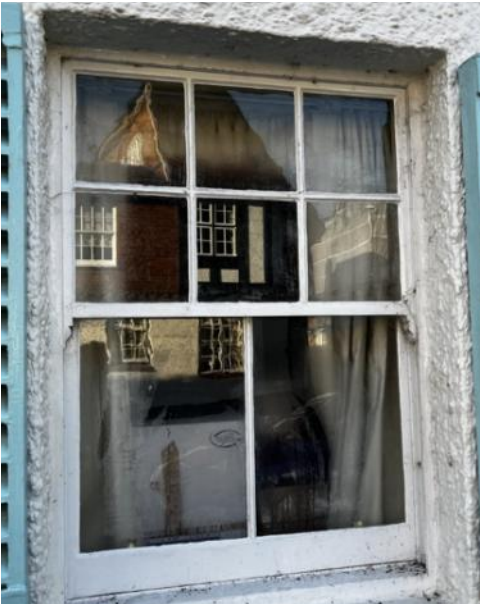
Existing timber sash windows
