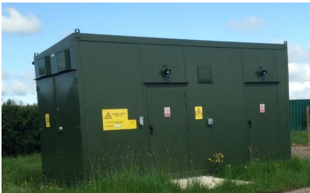
Plate 1: Example of a substation in Holly Green finish.
