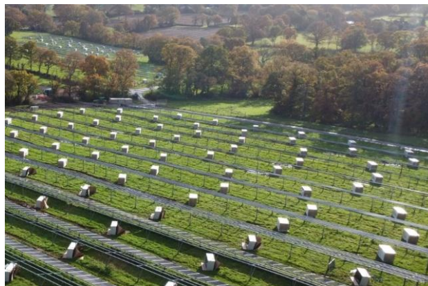
Examples of solar panels stacked ready for installation onto framework.
