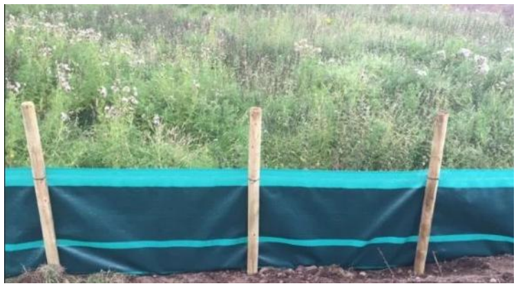
Perimeter fencing will be installed as the first stage of work. Example of silt fence.
