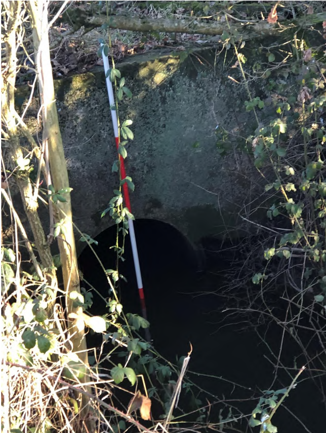
Figure 7 – Ordinary Watercourse Central Crossing
