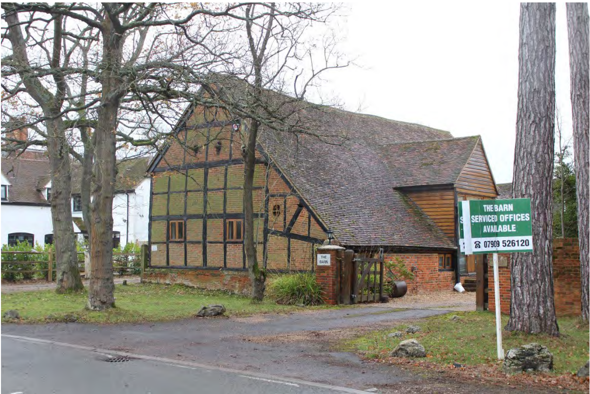
Image EDP A1.5: View of Grade II Lock's Barn ( 1135838 ) facing south-east.
