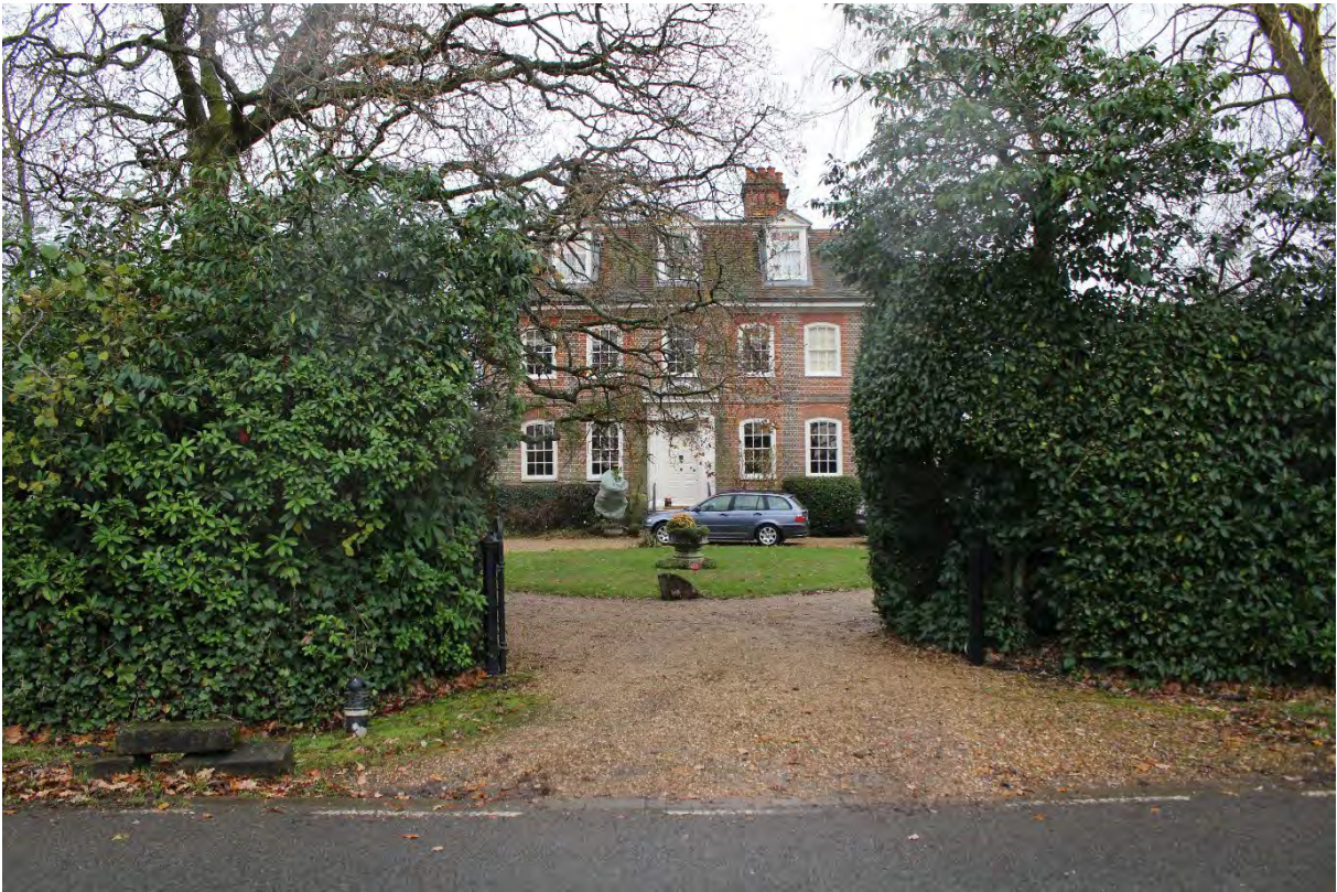
Image EDP A1.4: Main elevation of Grade II* Lock's House ( 1118082 ) facing south.
