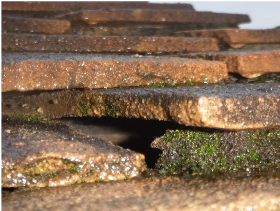
Photograph 3. No signs of recent or historic use of features by roosting bats (front elevation).
