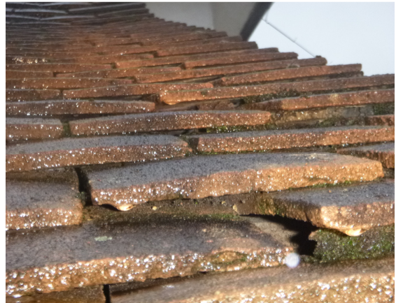
Photograph 4. No signs of recent or historic use of features by roosting bats (front elevation).
