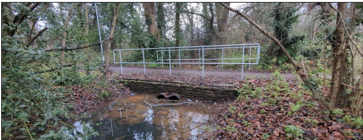
Figure 3: Existing culverted crossing on site.
