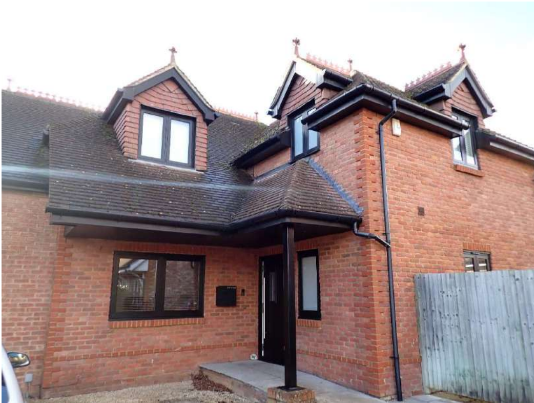
Photograph 1 – Southeast aspect of the building.
