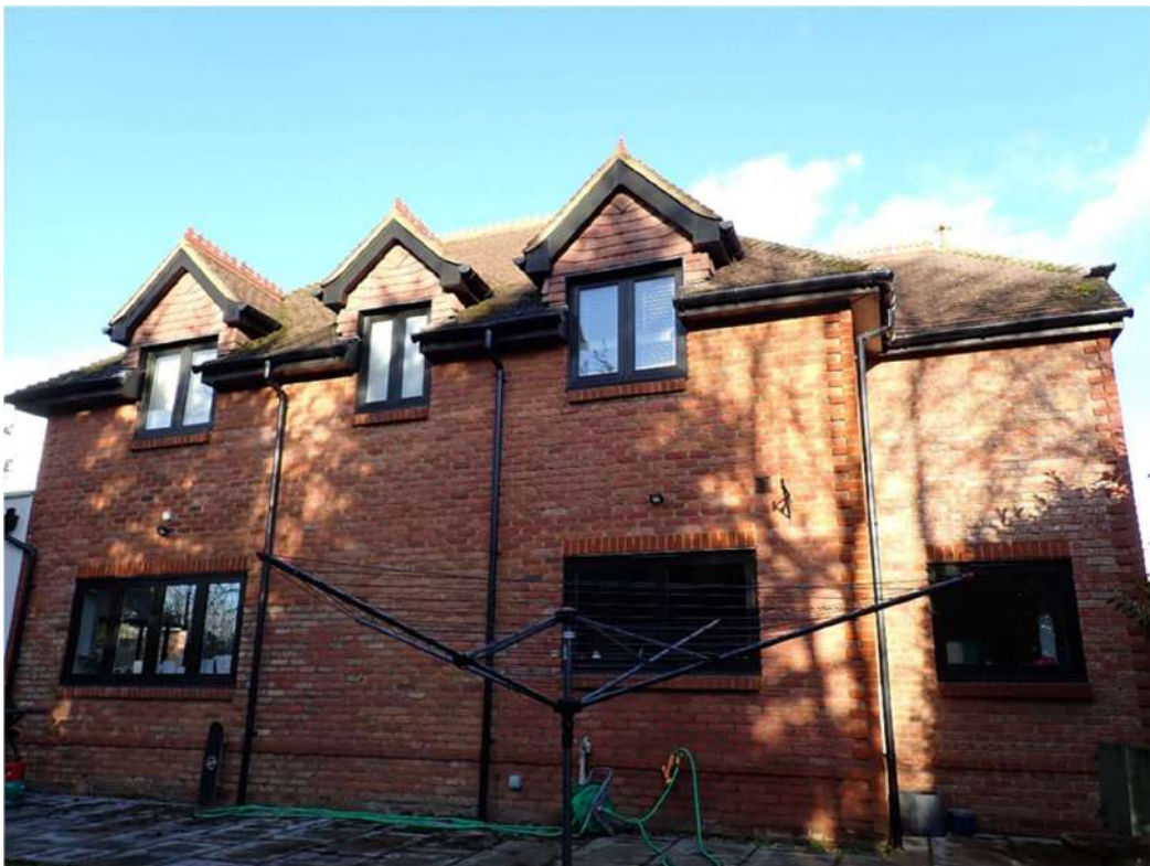
Photograph 2 – Western Aspect of the building.
