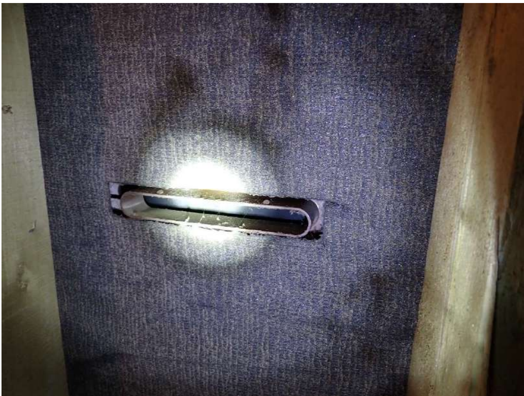
Photograph 16 – Ventilation slit which may provide a potential access point into the loft.
