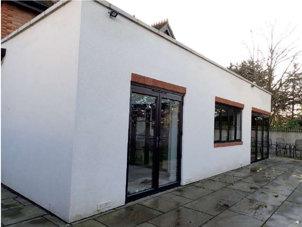
Photograph 13 – Single storey extension present on northern aspect of the building.
