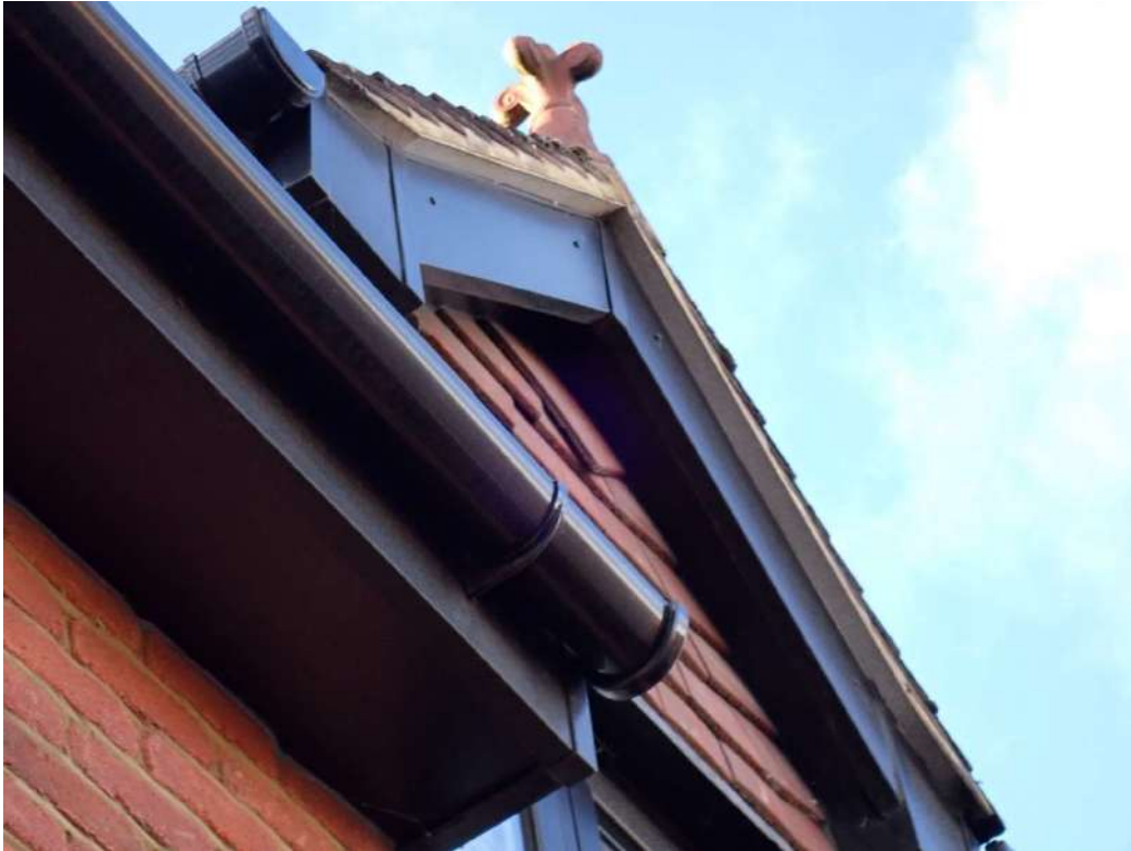
Photograph 9 – Raised end tiles on northeastern dormer.
