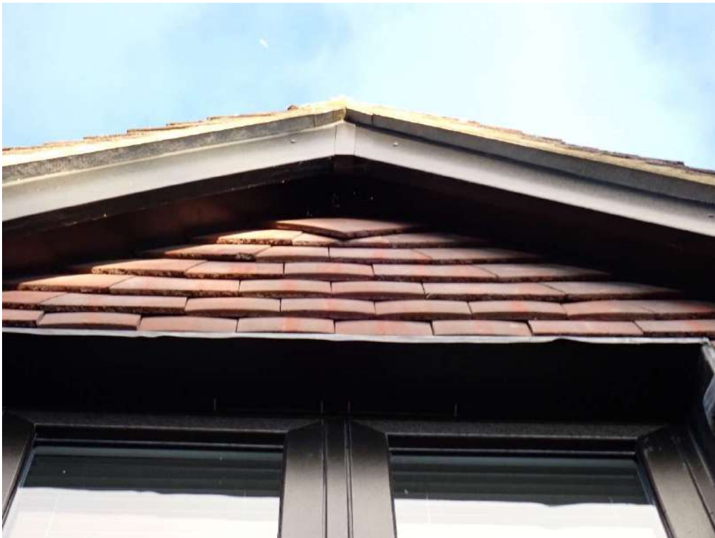
Photograph 6 – Well sealed boxed soffits on the dormers.
