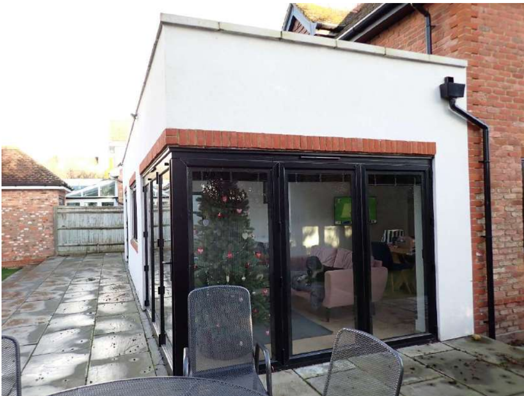
Photograph 14 – Single-story extension on northern aspect of the building.
