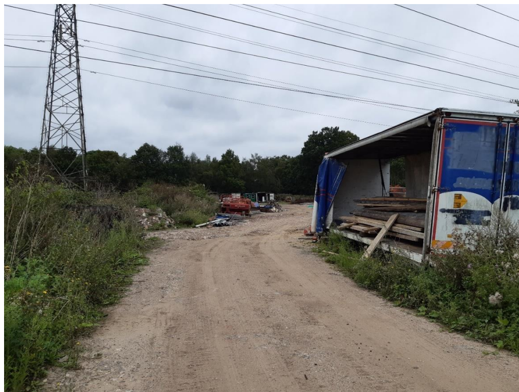
Figure 6: Case Officer site visit photo (dated 17 th August 2021) showing the left side of the field cleared of storage.
