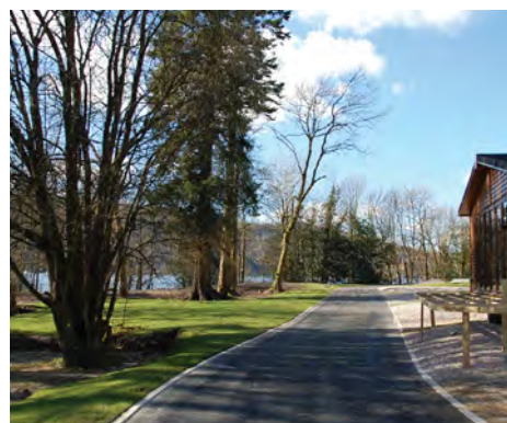
Fallbarrow Park, Windermere: Completed CellWeb TRP® Installation
