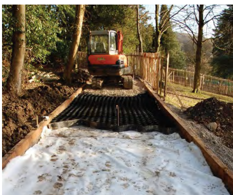
Fallbarrow Park, Windermere: CellWeb TRP® Installation
