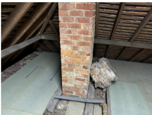
Photograph 5. The loft space of the building.
