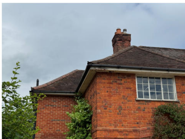
Photograph 4. The building viewed from the south-west.
