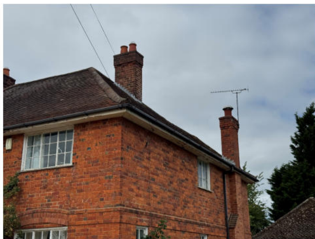
Photograph 2. The building viewed from the south-east.
