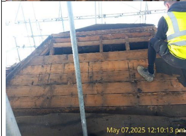
Figure 6: The upper most small, pitched clay-clad roof was also stripped under supervision.
