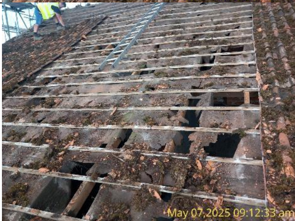
Figure 4: Roof during the licensable works.
