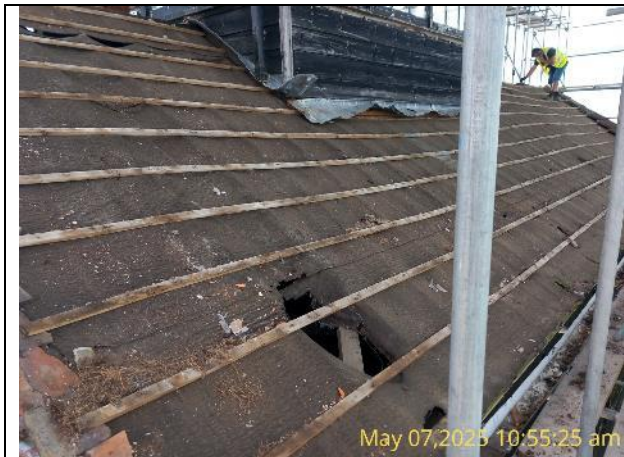
Figure 5: Roof after the licensable works.
