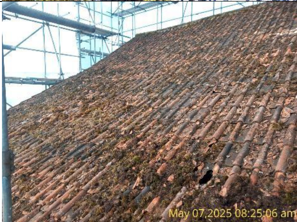
Figure 3: Roof prior to licensable works.
