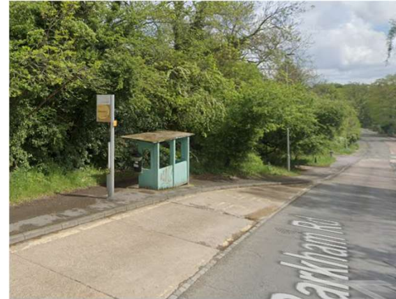
(i) Bus Stop directly outside the site
