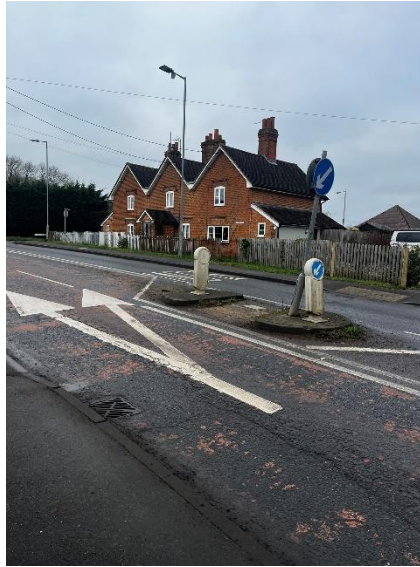
Photograph 3: Pedestrian Crossing on Barkham Road
