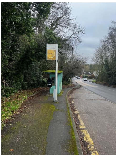
Photograph 4: Bearwood Road bus stop
