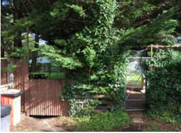
7. Poor quality landscape and boundary treatment
