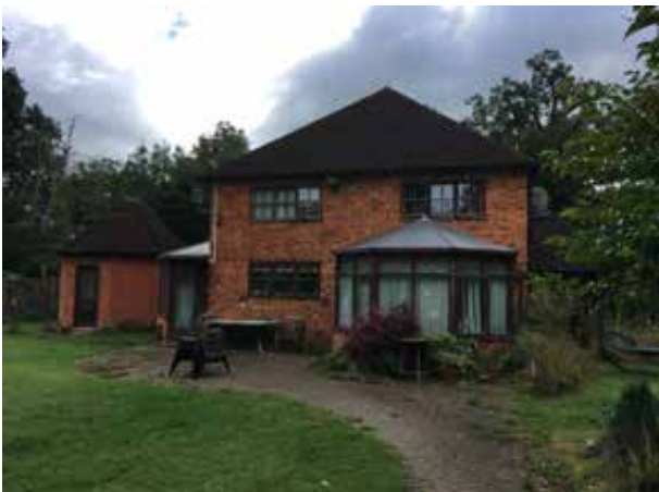
1. Rear (west) of Dairy Cottage
