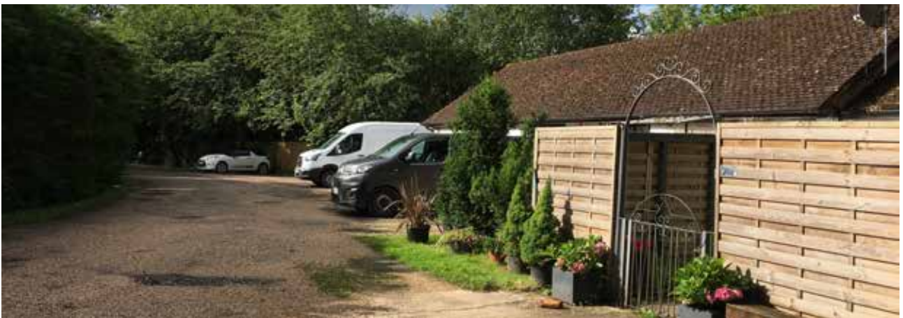
10. Lawful dwellings along the western boundary
