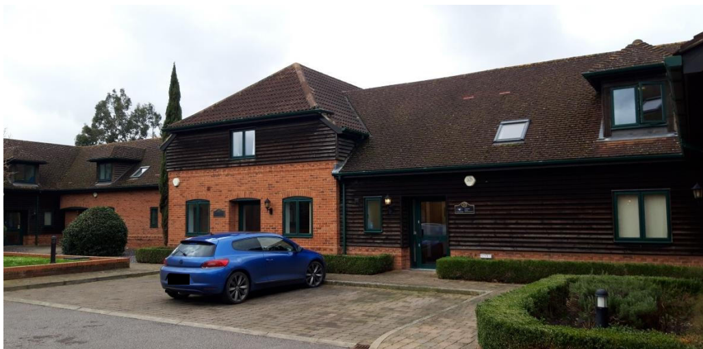
Traditional materials and rural architectural style of existing main building
