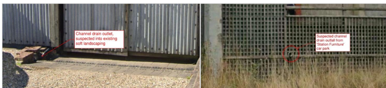
Figure 2.4: Existing surface water drainage outfalling into undeveloped land on-site.
