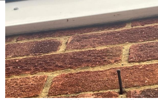
Figure 4: Tightfitting against wall
