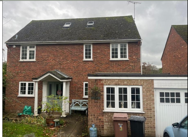
Figure 1: The front elevation and garage of B1
