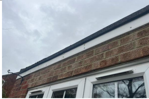
Figure 3: Well sealed bitumen felt and uPVC
