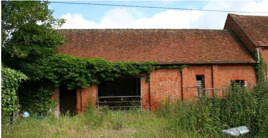
The southern elevation of the Brick Stables.
