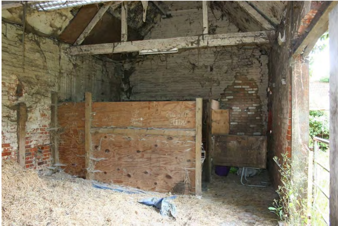
The stalls are made from LC20th materials.
