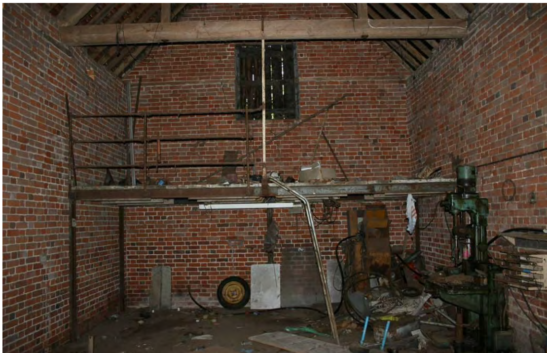
Looking E inside the Brick Barn.
