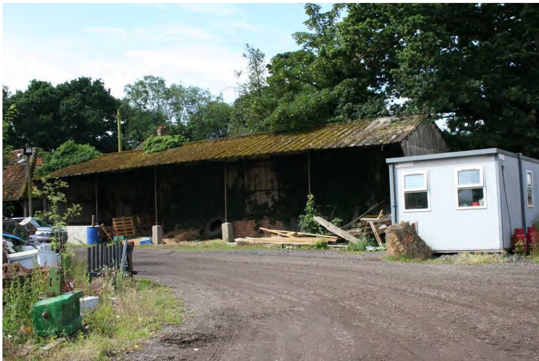
Hay Barn west of the farmyard. Looking SW.
