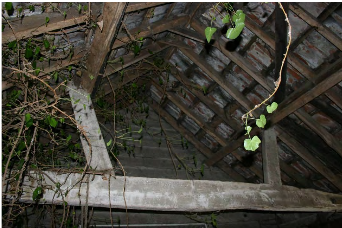
Looking E in the roof of the Garage Workshop.
