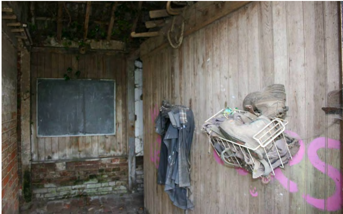
Entrance corridor with tongue and grooved boarded walls. Note the harness pegs.
