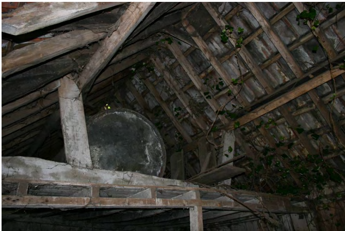
The roof of the Garage Workshop.
