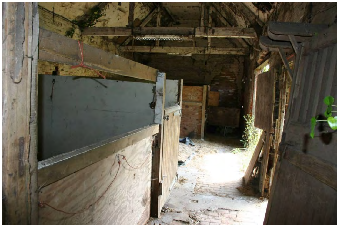
Looking E in the main stable.
