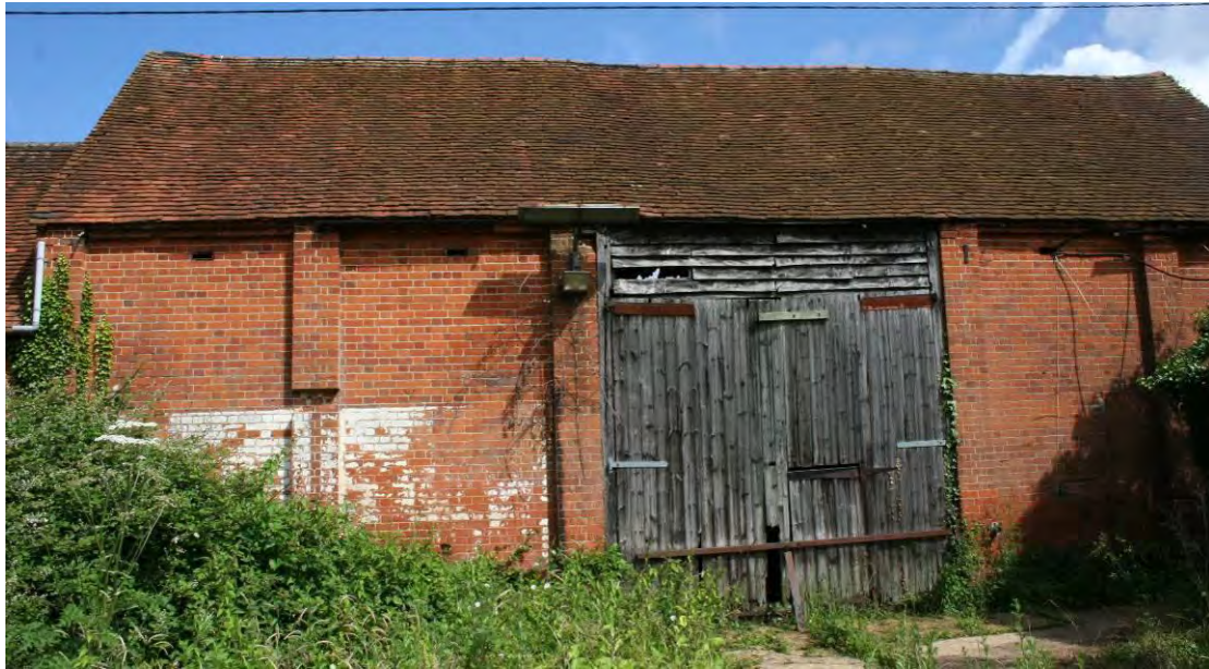
The southern elevation of the Brick Barn.
