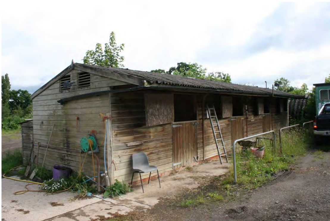
Working stable block north of the farmyard. Looking NE.
