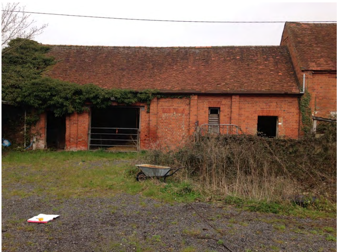
BUILDINGS 'D' & 'E'
