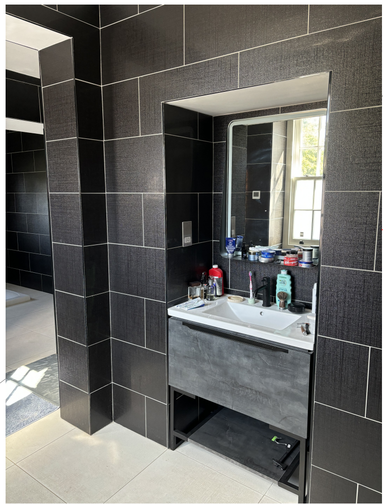
View from bathroom - existing modern timber stud partition removed to unblock opening
