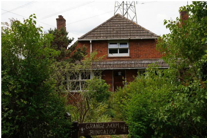
P6 Grange Farm Bungalow Photo 1 - View north west from main entrance
