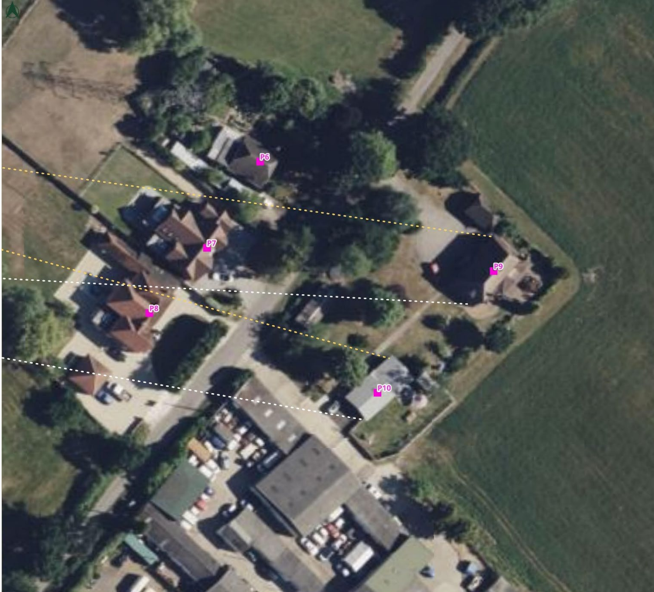
P9 Grange Farm and P10 Stable View – Aerial View
