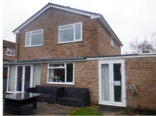
Photograph 2. Rear of the house viewed from the south.
