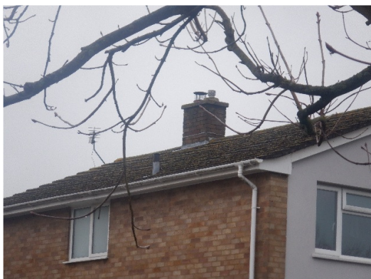
Photograph 7. Tight lead flashing around the chimney and flue pipe.
