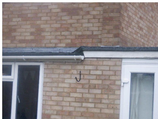
Photograph 9. Tightly fitted roof on the rear extension.
