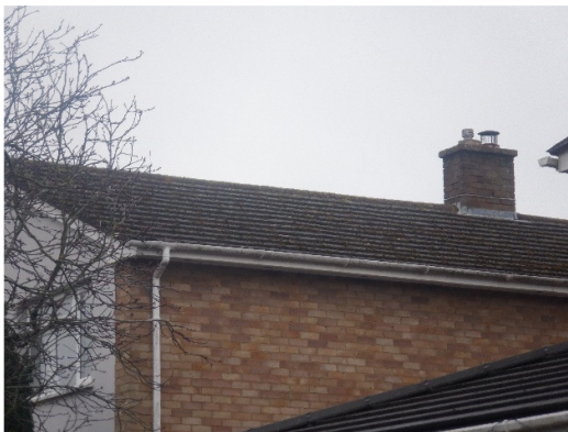
Photograph 3. Flat and intact roof tiles.
