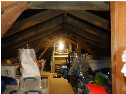
Photograph 10. Internal view of the roof void.
