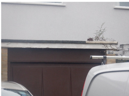
Photograph 8. Tightly fitted roof on the garage.
