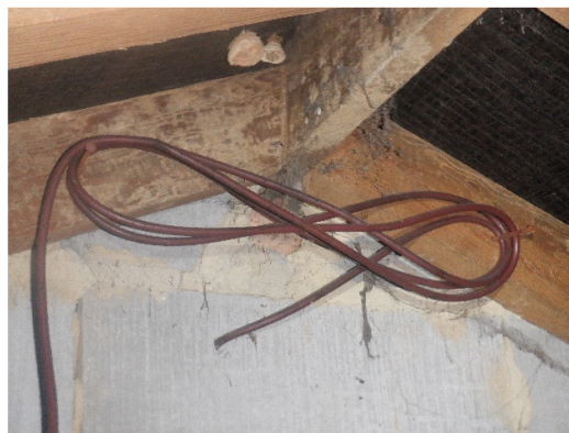
Photograph 15. Tight and heavily cobwebbed blockwork gable end.
