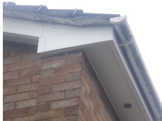
Photograph 4. Soffits tight to the eaves.
