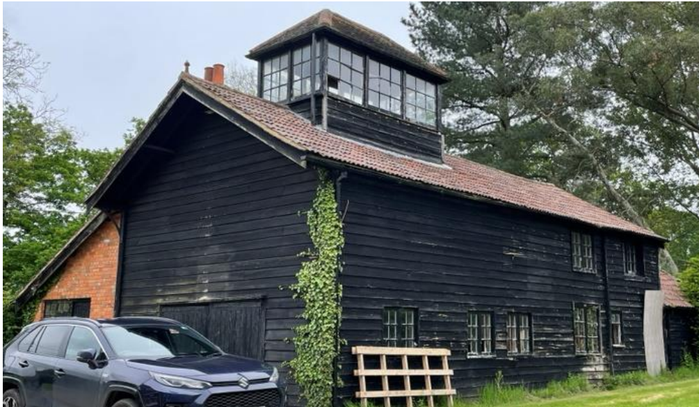
Photo 1: the southern and western elevations of B1.
