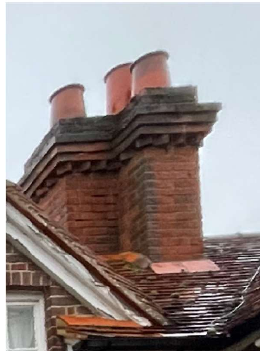
Tiled Roofs / Brick Chimneys / Flues
