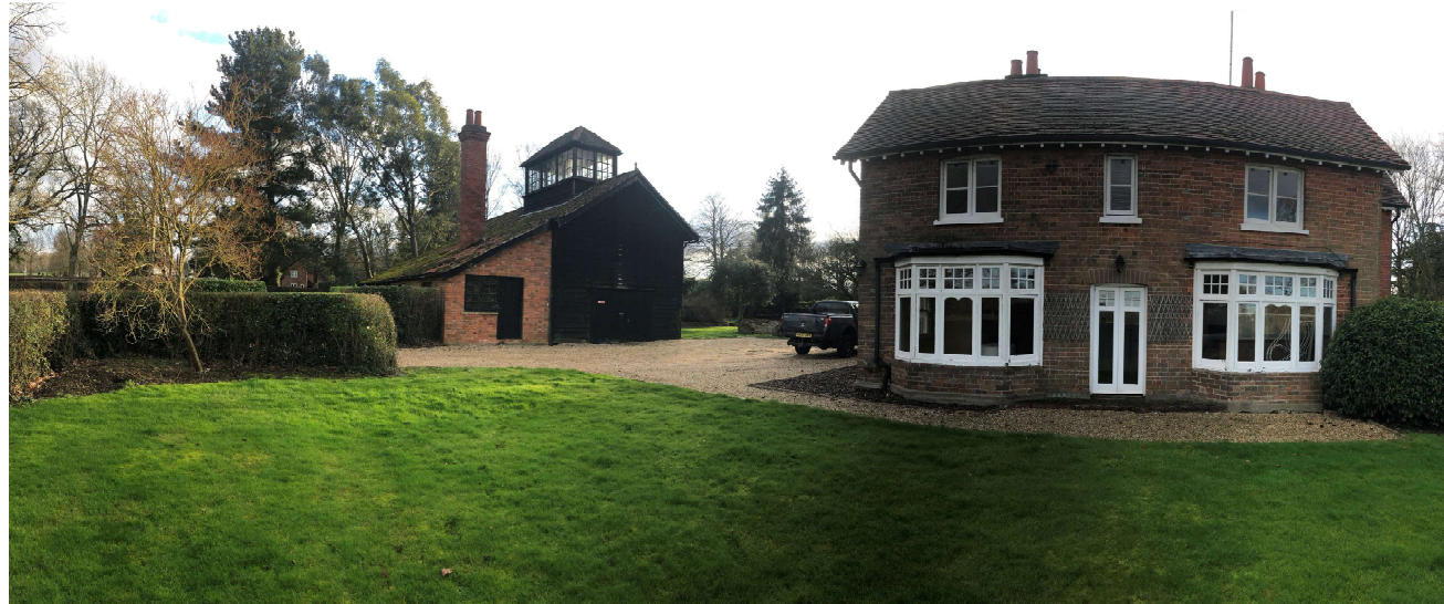
Existing View From North East
