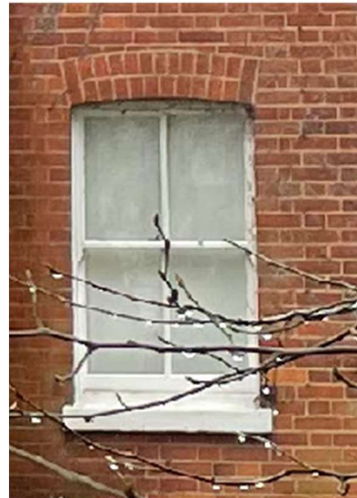
Stone Window Sills / Brick Lintels
