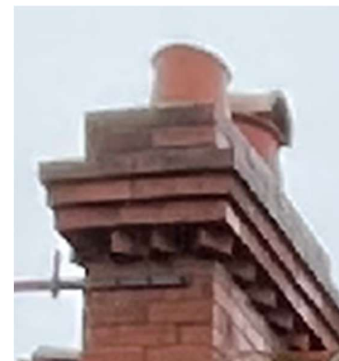
Red Brick Chimneys / Terracotta Flues
