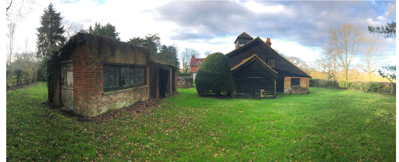
Existing View From South East
