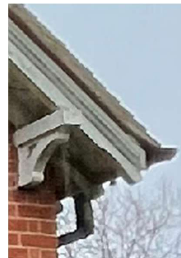
Roof Facias & Eaves
