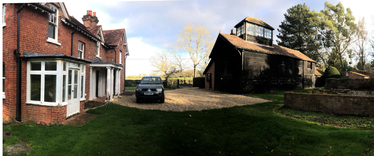
Existing View From South
