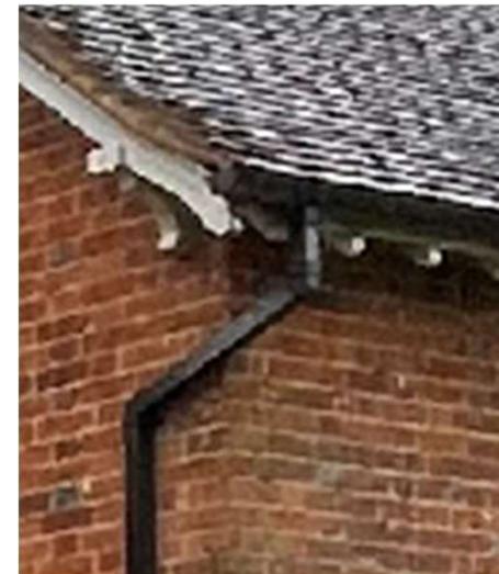
Cast Iron Rain Water Pips
