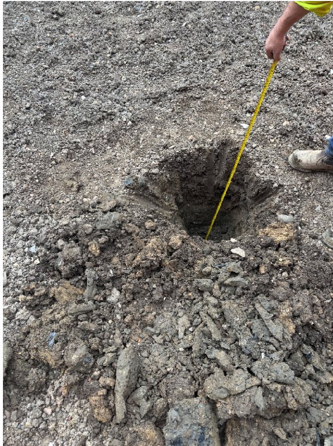
Inspection Pit excavated by client in Plot 133 (client-provided photograph)
