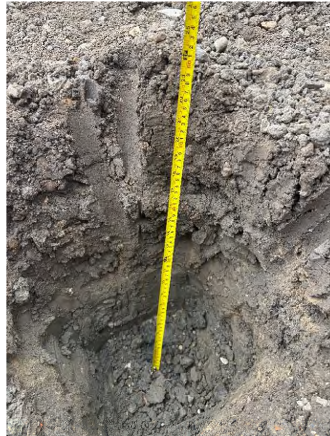
Inspection Pit excavated by client in Plot 133 showing 600mm of clean cover (client-provided photograph)
